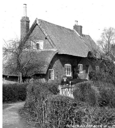
One of the Well head cottages in Stretton
